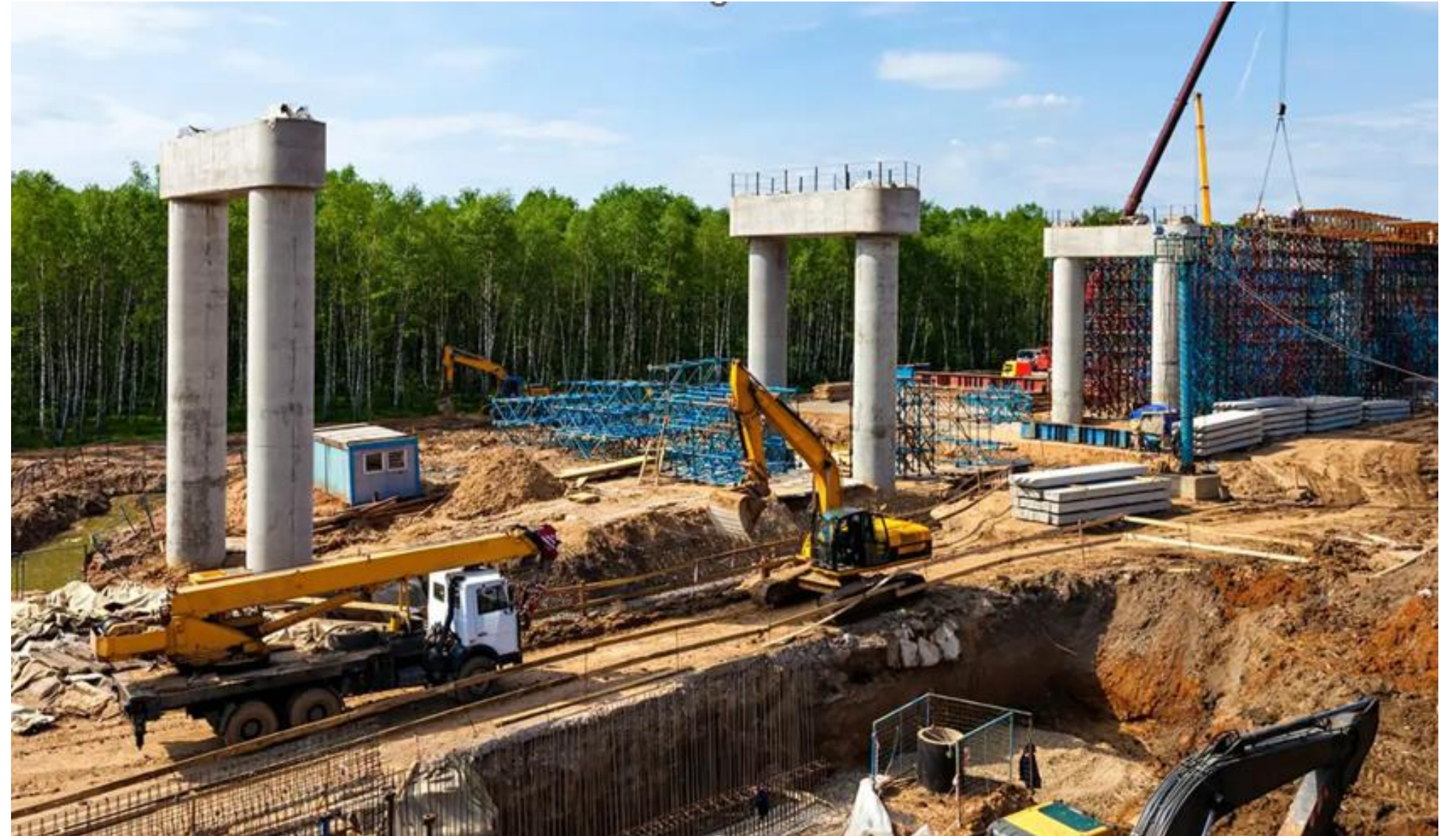
Illustrative photo of bridge construction
